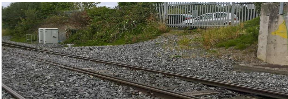
Figure 33 – Ballast Pad (for on-tracking & off-tracking RRVs)
