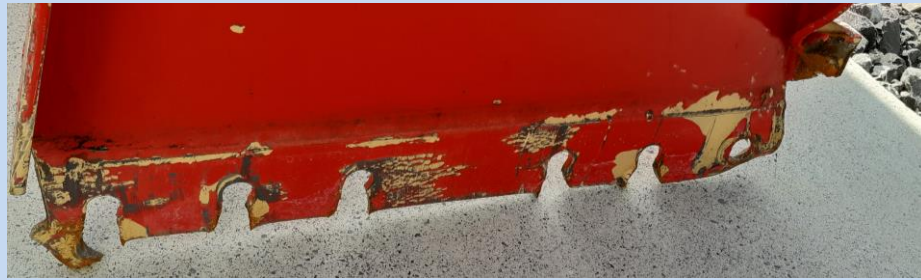
Photograph 1 – Image of buffer stop after accident:
