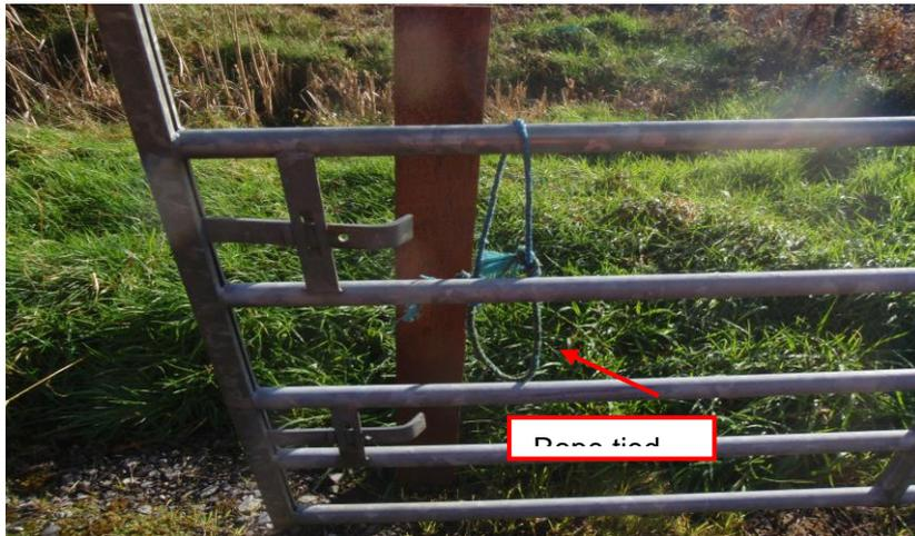
**Figure 25 – LC XM220 gates tied to keep level crossing open**
