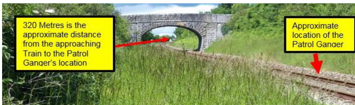
Figure 5 – Sighting distance, as calculated by IÉ-IM
