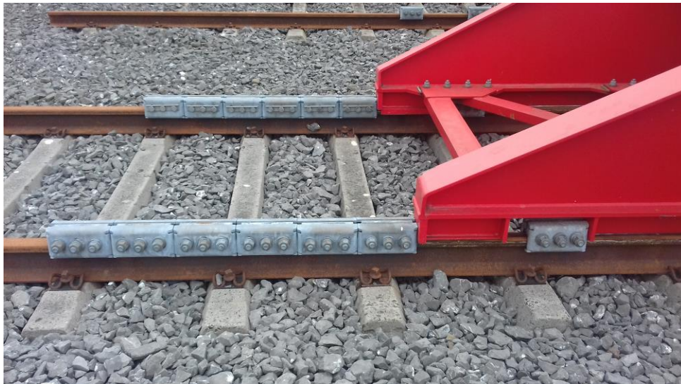
Figure 18 – Rawie buffer stop after the accident
