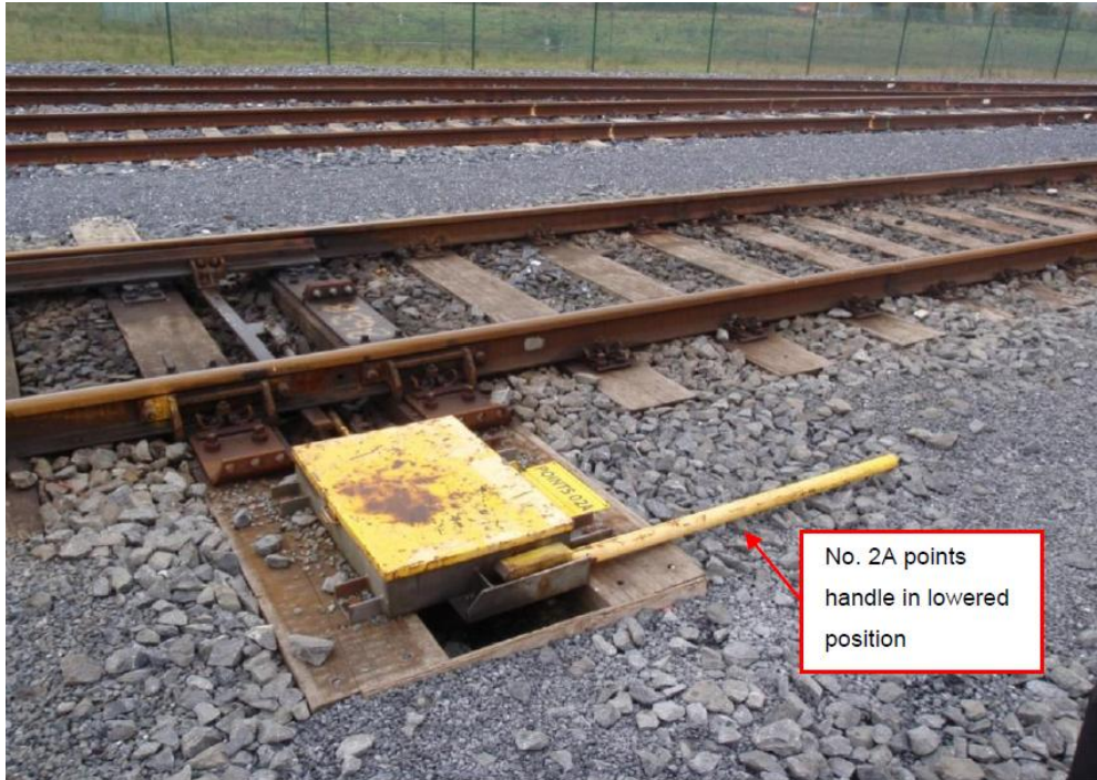
Photograph 3 – No. 2A points with points handle disengaged
