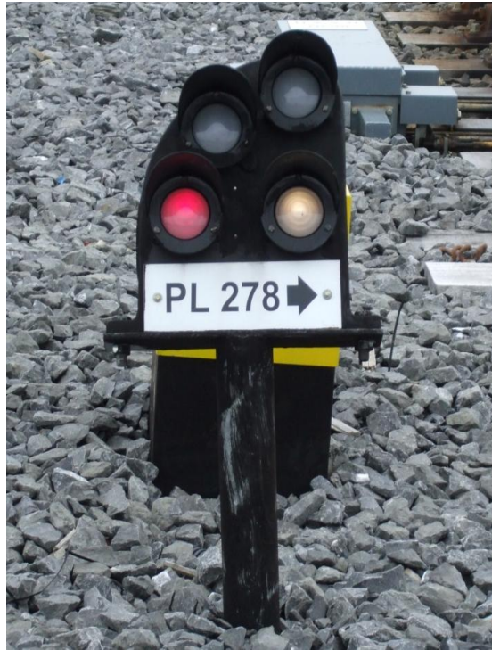
Photograph 2 - Signal PL278 illuminated by filament lamps
