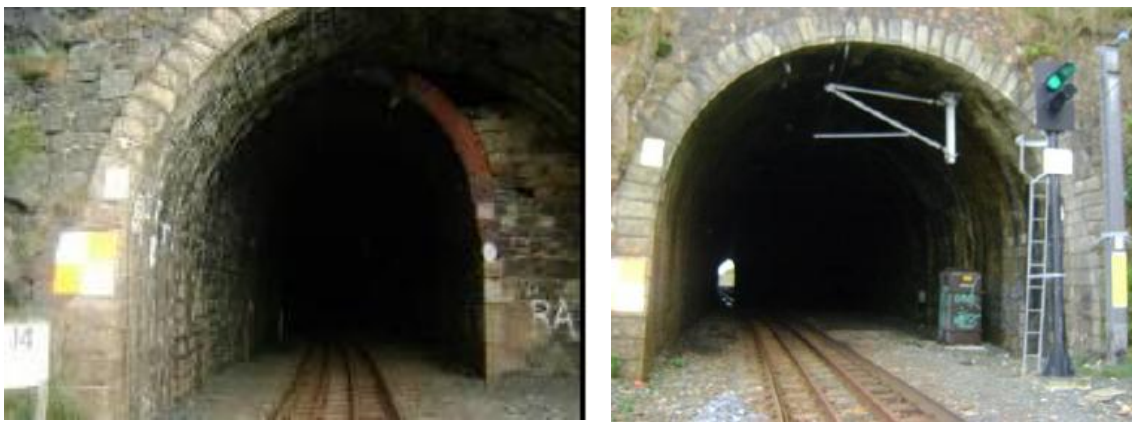
Figure 6 – Tunnel No. 2 portals (note the difference in bore widths)
