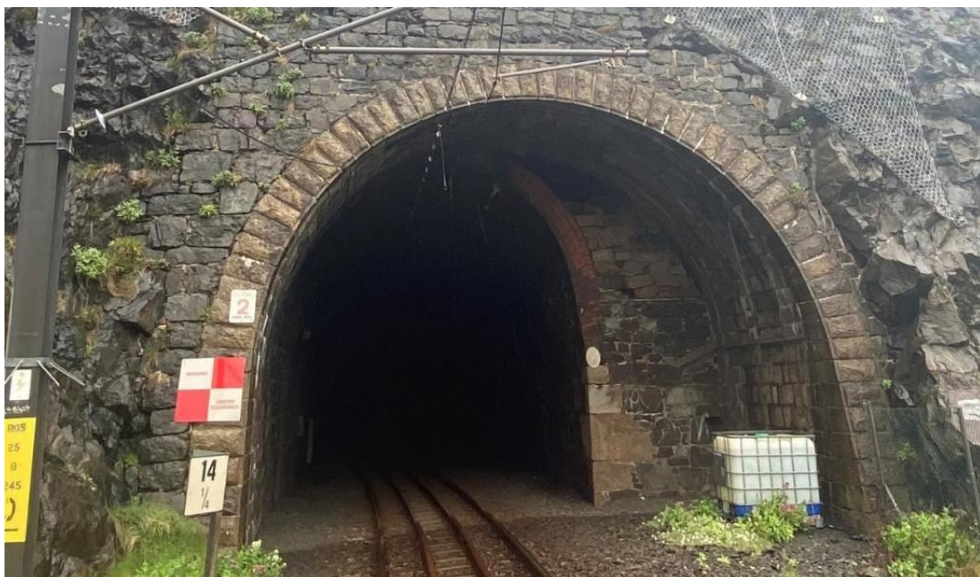
Figure 2 – Bray Tunnel No. 2 viewed from the southern portal
