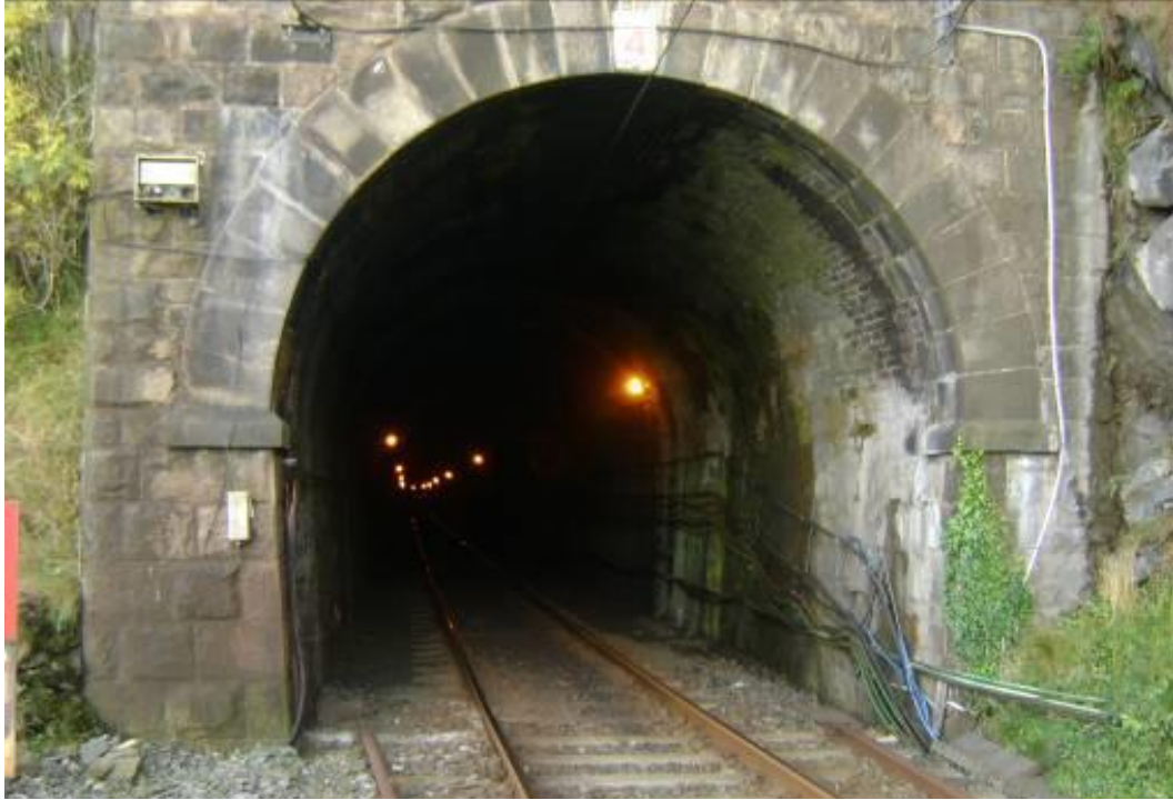
Figure 3 – Bray Tunnel No. 4
