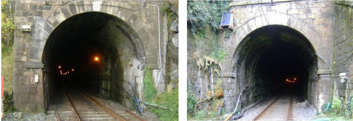
Figure 7 – Tunnel No. 4 portals
