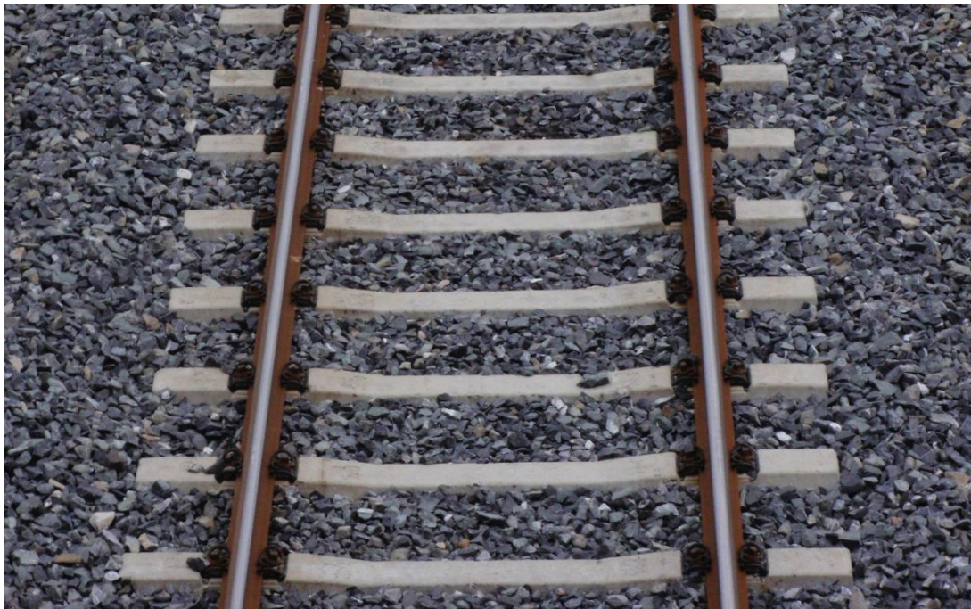
Figure 3 – Flat bottom track as installed at the location
