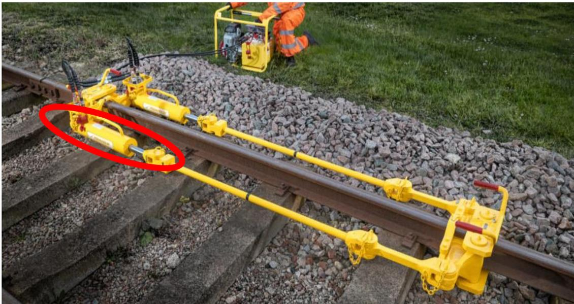
Figure 5 – Rail Tensors attached to rail
