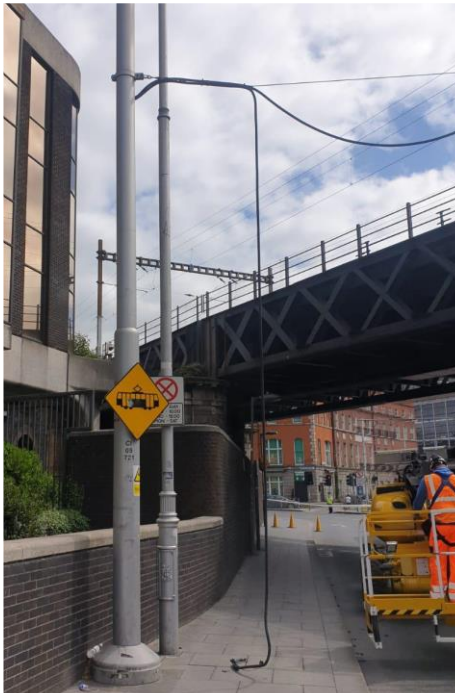
Figure 19 – Feeder cable down
