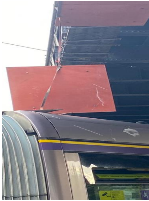
Figure 20 – Damage to insulated plates
