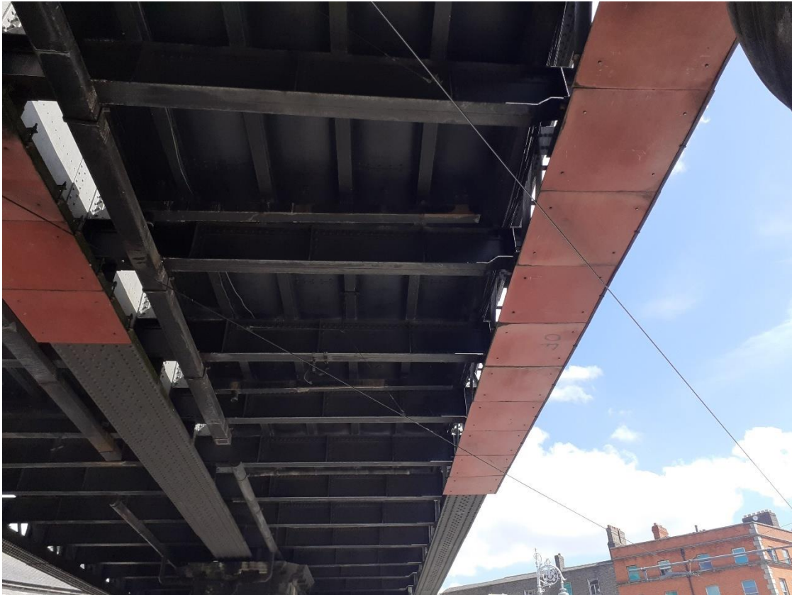
Figure 11 – Insulated plates under Beresford Place railway bridge
