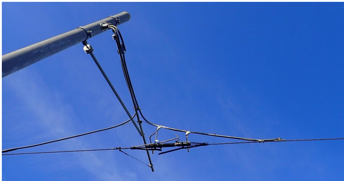
Figure 4 – Section Insulators on the OCS
