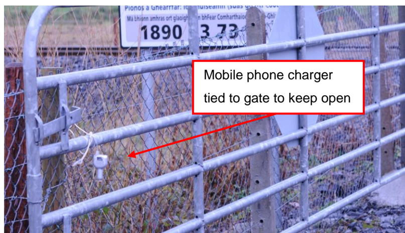
Figure 22 – Gates tied open with mobile phone charger
