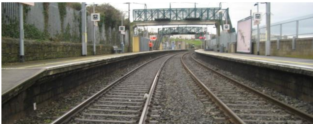
Figure 2 – Salthill & Monkstown Station (southbound track on right)
