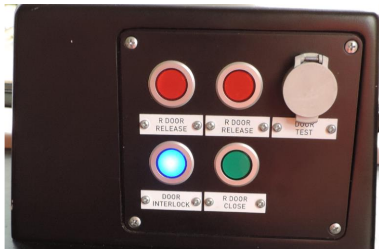
Figure 14 – Driver's control panel for right hand side door operation controls
