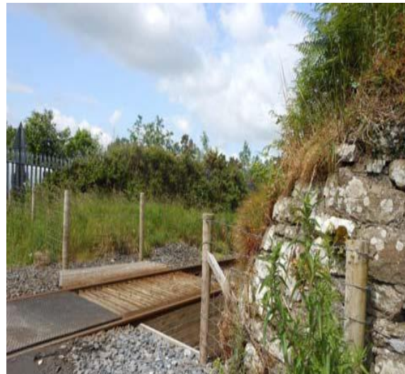
Figure 8 – View on Up Side looking Down
