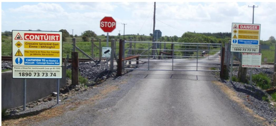
Photograph 2 – Typical user worked level crossing on the IÉ network
