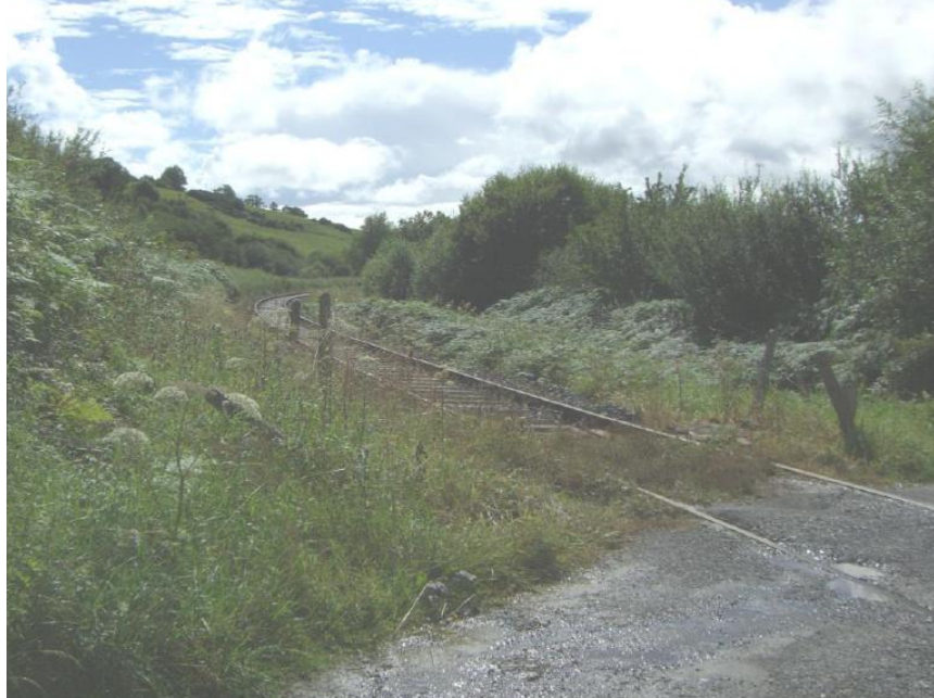
Photograph 5: View from Cappadine level crossing
