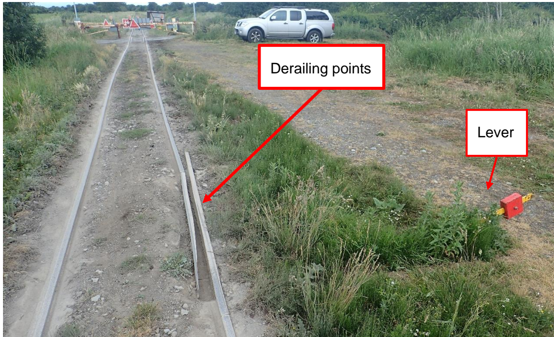
Figure 6 – Derailing points (in the open position – locomotive would derail)
