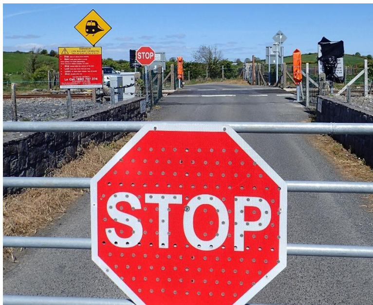
Figure 12 – Examples of Warning Signs at the approach to and at LC XM240
