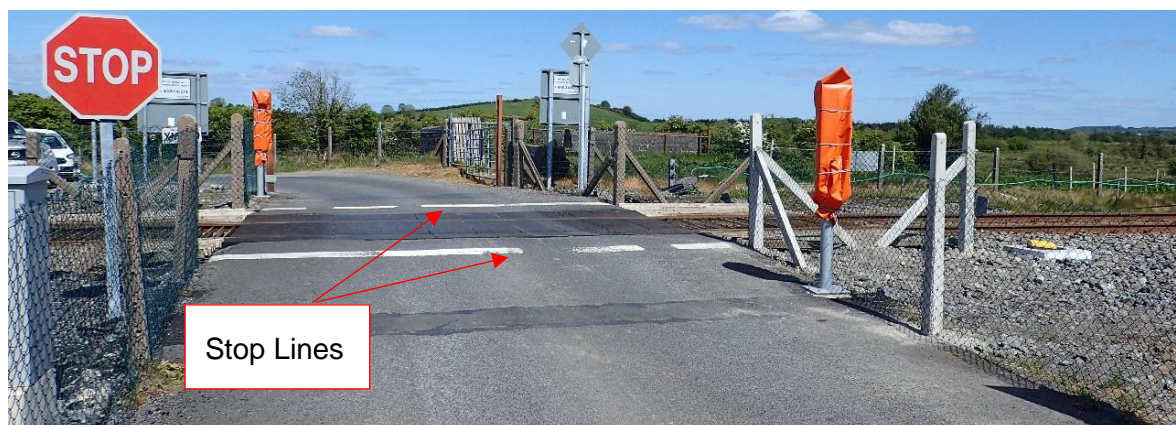
Figure 14 – LC XM240 Stop Lines on either side of the railway
