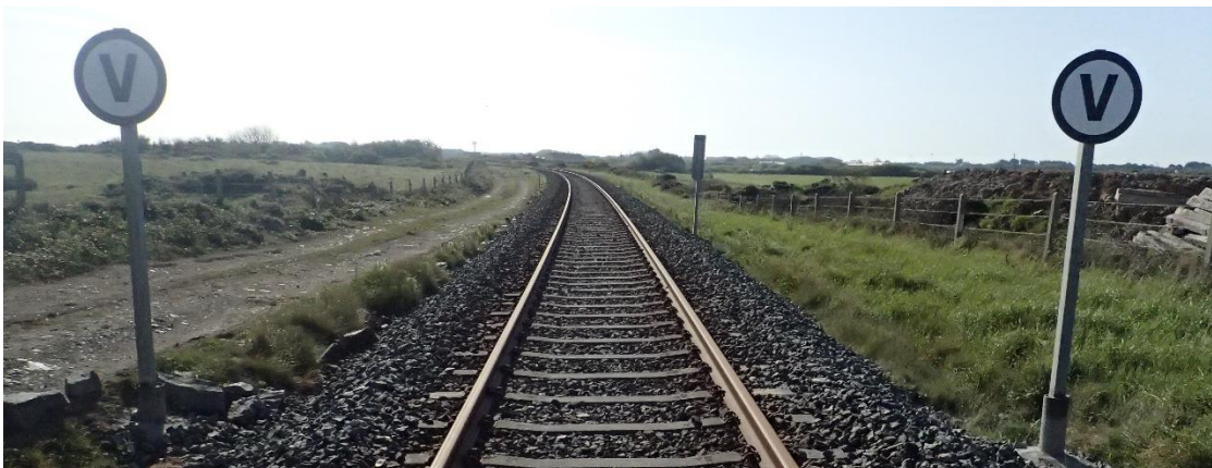
Figure 5 – Photograph of V Boards taken, when erected, after the accident
