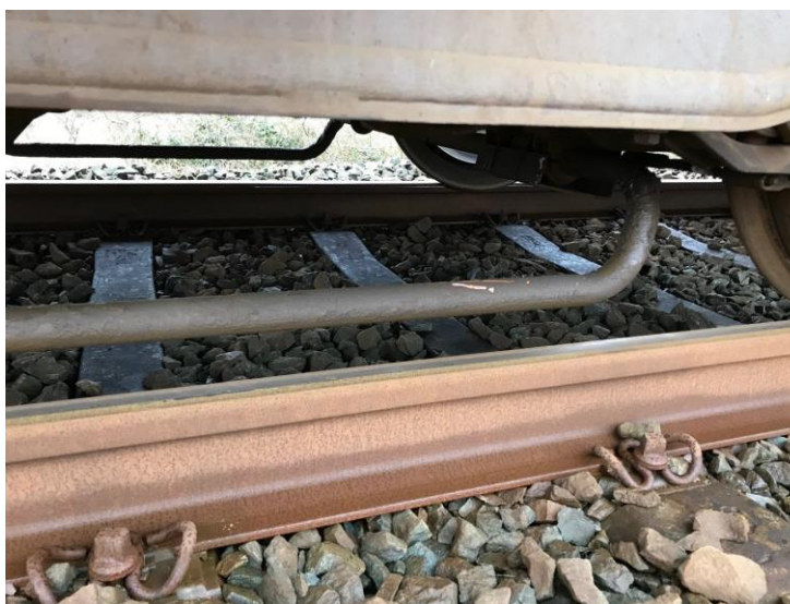
Figure 3 – Damage to TCA on ICR 22343
