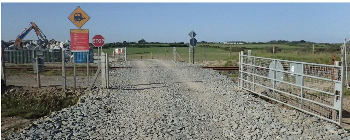
Figure 4 – Level Crossing XR102
