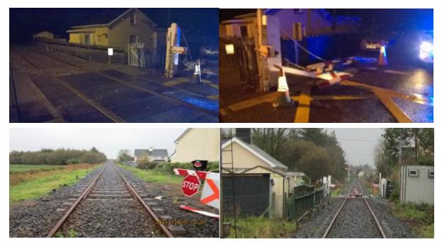
Figure 22 – Damage to gates at Level Crossing XN159 Spa
