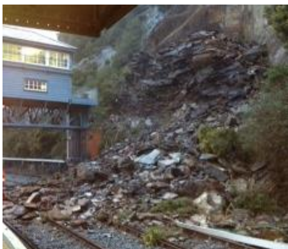
Figure 7 Landslide obstructing track
