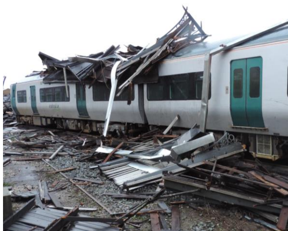
Figure 6 Debris on train at Cork station
