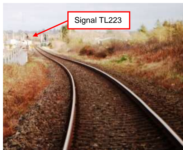
Figure 23 – View of Signal TL223 on curve
