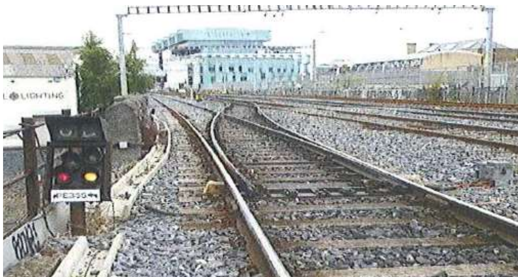
Figure 86 – Position light signal, Signal PE35s
