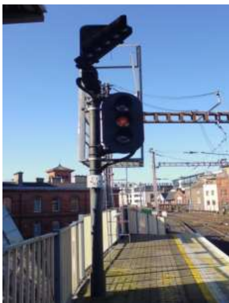
Figure 99 – Signal CY91 (Platform 5)
