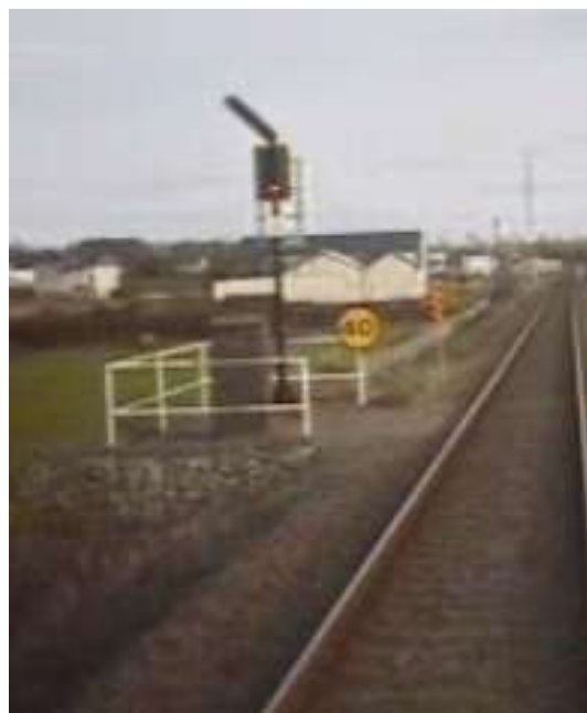
Figure 26 – Train A303 CCTV download, showing Signal TL223 displaying a red aspect and speed board
