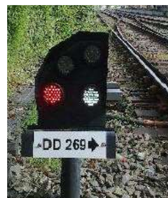
Figure 92 – Shunt Signal DD269
