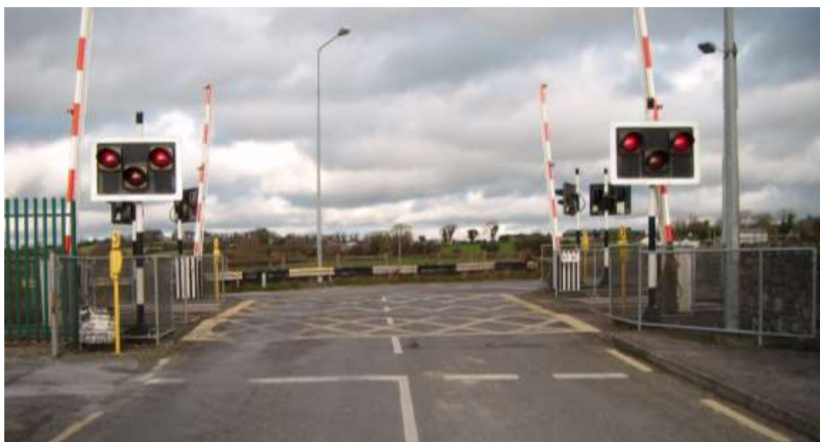
Figure 21 – Level Crossing XT061
