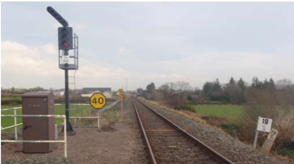
Figure 22 – Signal TL223 with route indicator and adjacent speed board
