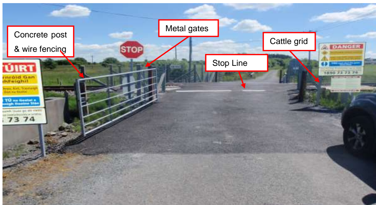
Figure 9 – Features of the level crossing
