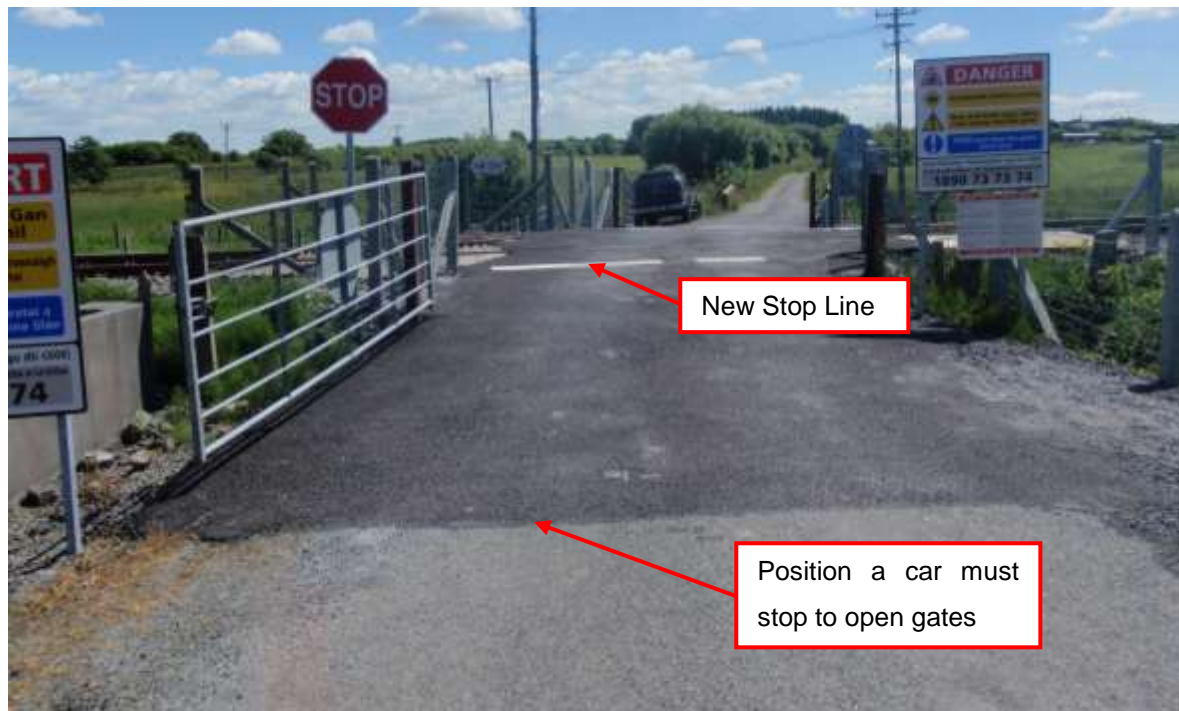
Figure 28 – Car Driver's stopping position and New Stop Line stopping position
