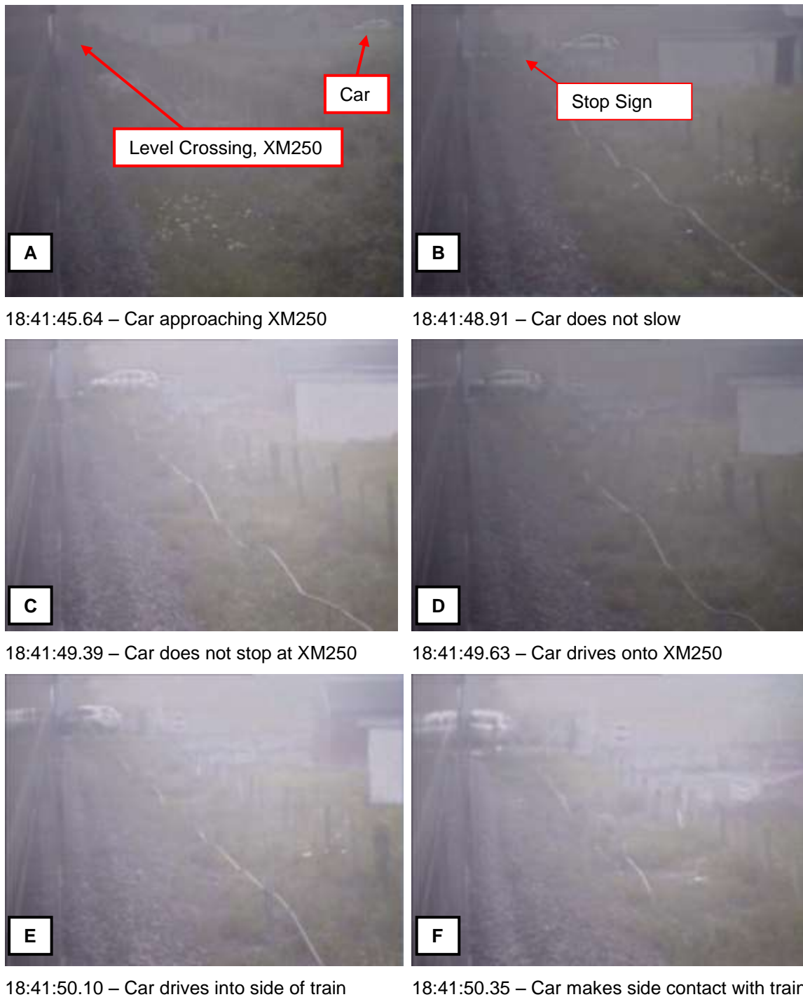
Figure 2 – Car approaching Level Crossing and striking train
