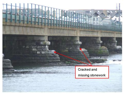
Photograph 15 – Photograph taken by the AE on the 18<sup>th</sup> August 2009, showing defects to piers' stonework
