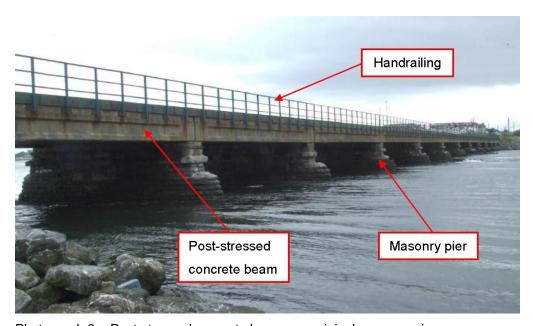
Photograph 3 – Post-stressed concrete beams on original masonry piers
