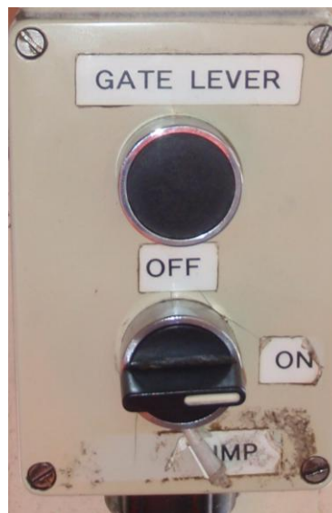
Photograph 5 – Gate Lever Lock
