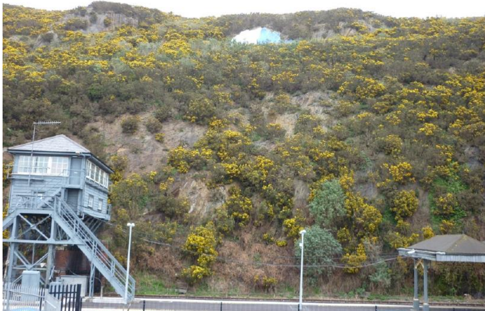
Figure 11 – Photograph taken in 2012, in the location of the 2013 rock fall
