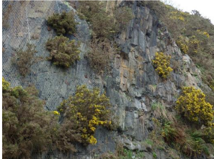
Figure 12 – Rock netting present in 2012 GEI
