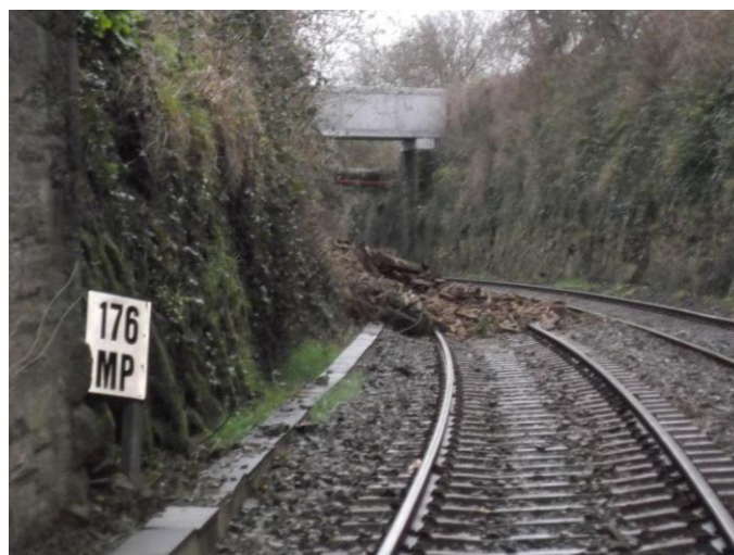
Figure 17 – Landslide at 176 MP
