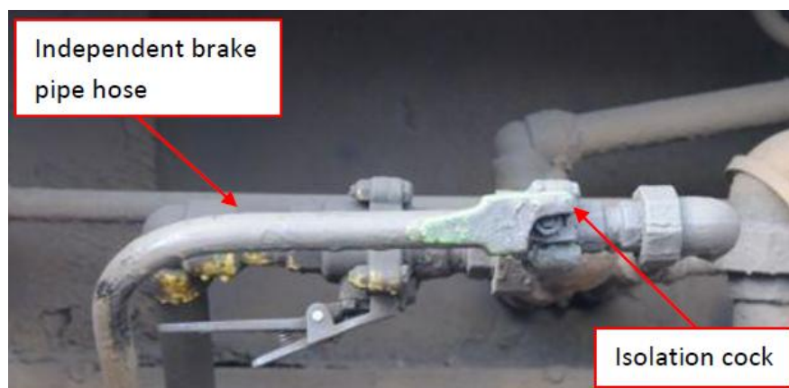
Figure 6 – Isolation cock for the independent brake pipe
