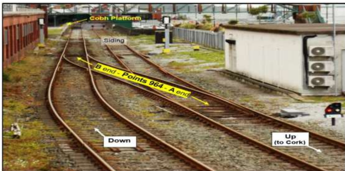
Figure 11 – Points 964 set to the normal position
