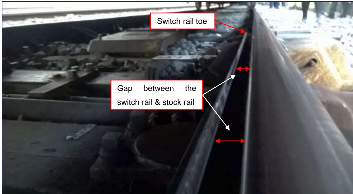
Figure 8 – Gap between the toe of the switch rail toe and the stock rail
